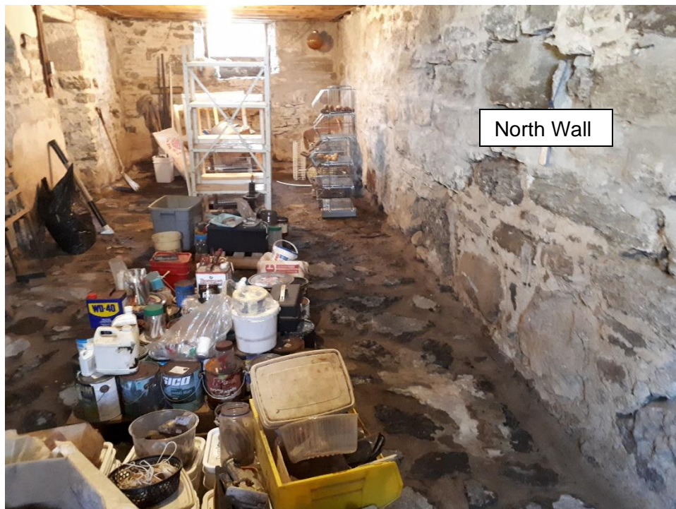
Figure 09 – Basement floor dry in Northern segment of basement.
