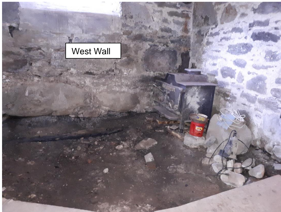
Figure 08 – Basement floor dry along West foundation wall.
